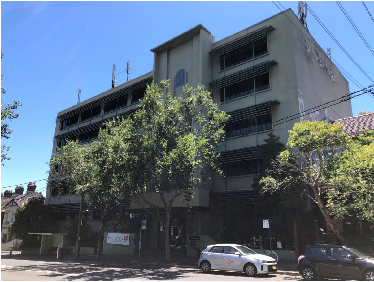
site viewed from Glebe Point Road
